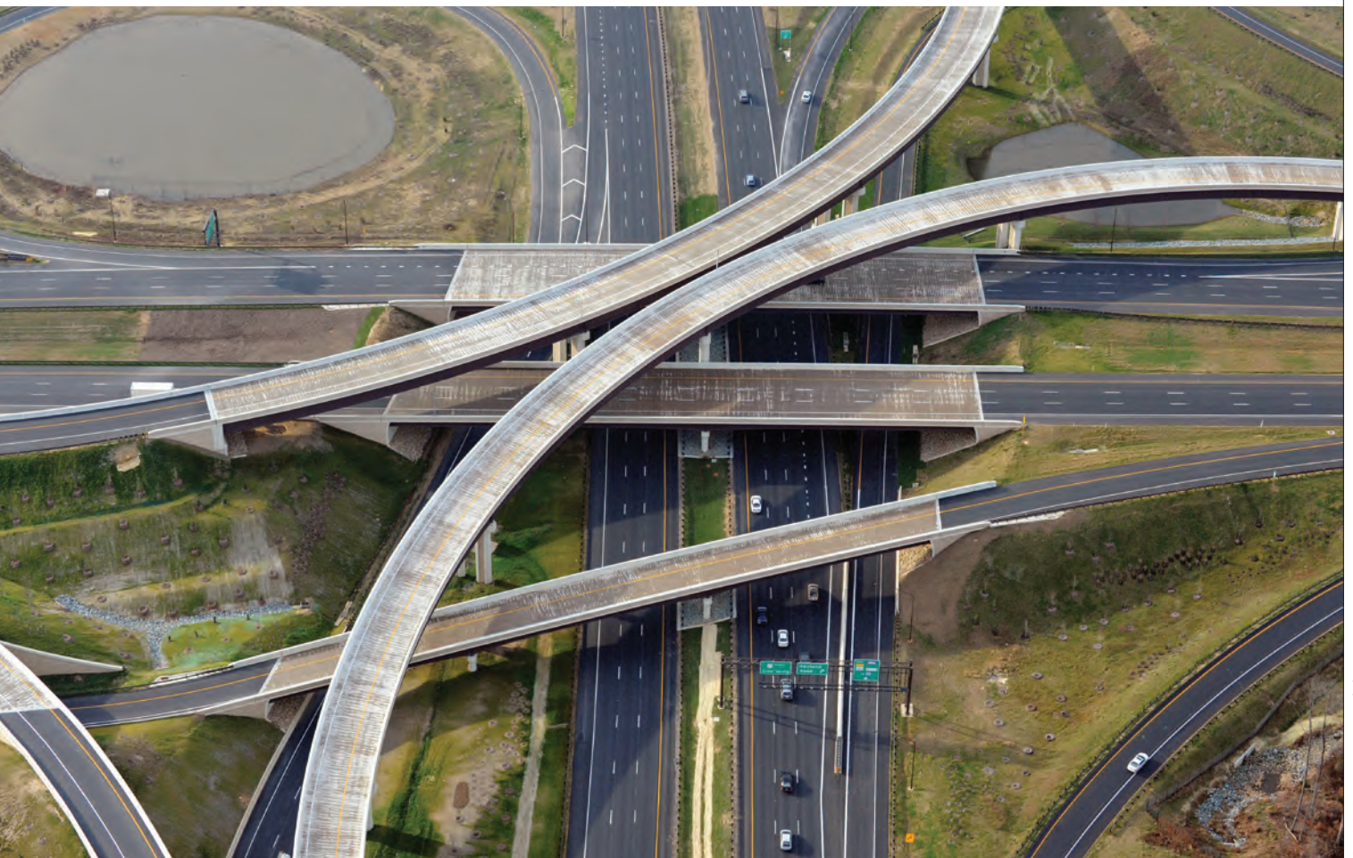
© ICC Constructors, a joint venture
